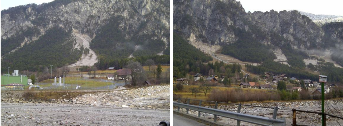
Figure 12 and 13. View of the three main debris channels that converge into the Fella river, one natural gas reserve and the other two surrounding the touristic village. December 2011.
