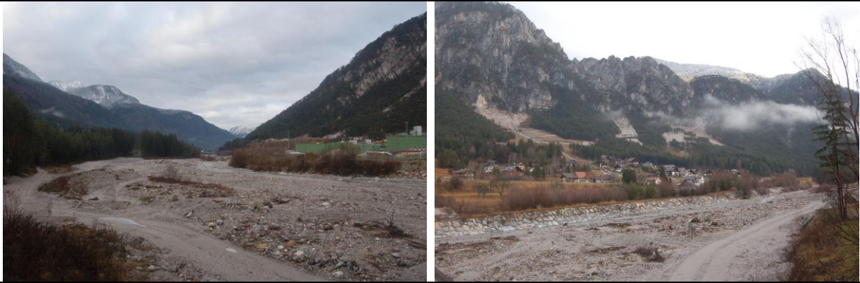
Figure 14 and 15. View of the Fella river upstream (left) and downstream (right) in which is evident the large amount of transported sediment that are visible due to the low water level conditions. December 2011.
