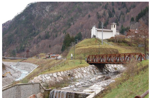
Figure 22 and 23. Upstream view of both sides of the river that covers the ongoing works for the protection of the piles and finilised works on the right side for the protection of the slope channel, disipation of energy and debris retention. December 2011.
