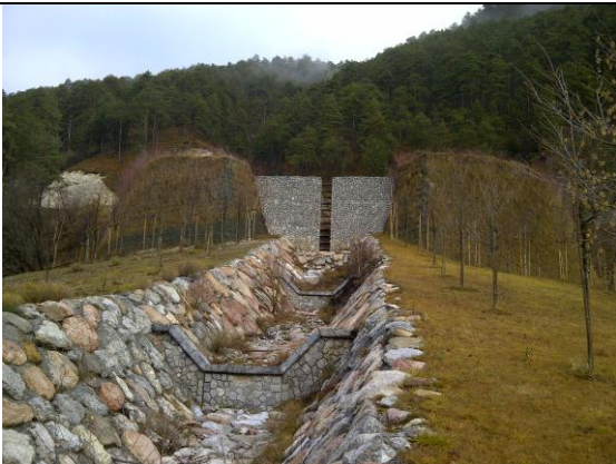
Figure 10 and 11. Overview of the hydraulic structure and the debris dam in which it can be appreciated the high slope of the terrain. Upstream the dam the channel is long enough to accumulate and important load of sediments that are temporary stored and later released when the tailwater is deficient of area sediments. It requires regular maintenance works after after medium and large size events. December 2011.
