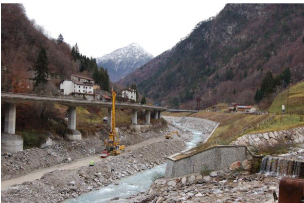
Figure 22 and 23. Upstream view of both sides of the river that covers the ongoing works for the protection of the piles and finilised works on the right side for the protection of the slope channel, disipation of energy and debris retention. December 2011.
