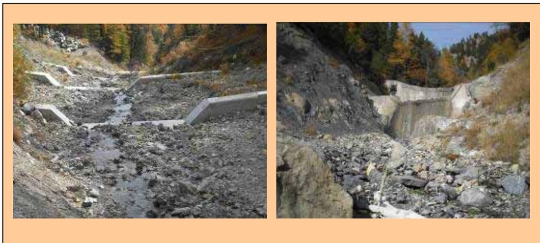
**Figure 9.** Check dams built in the Faucon basin
