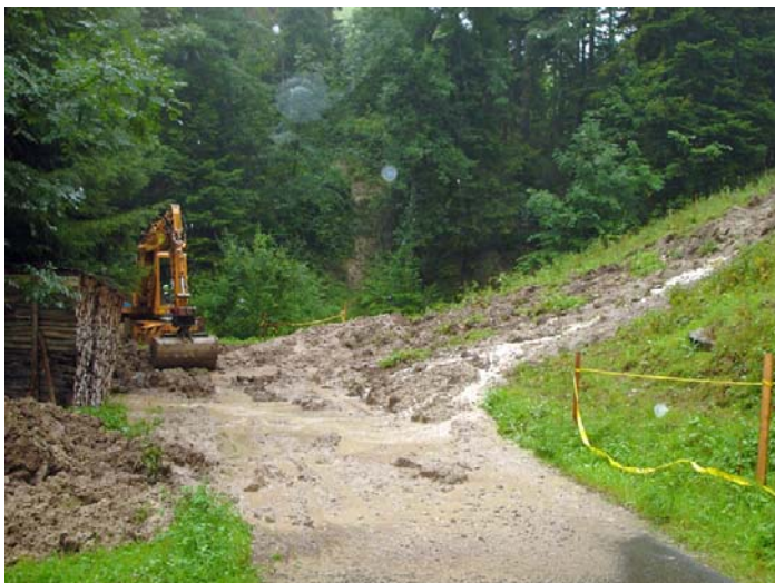
Figure 1: Exemplary road blocked by landslides.
