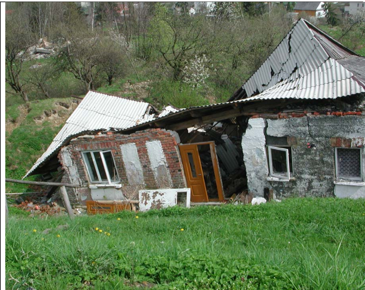
Photo 2. Landslide in Lachowice (spring 2002) - damaged houses (courtesy of W. Rączkowski, PGI)
