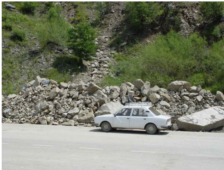
Rockfalls along Siriu reservoir and national road 10
