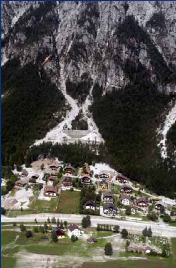
Before the intervention
