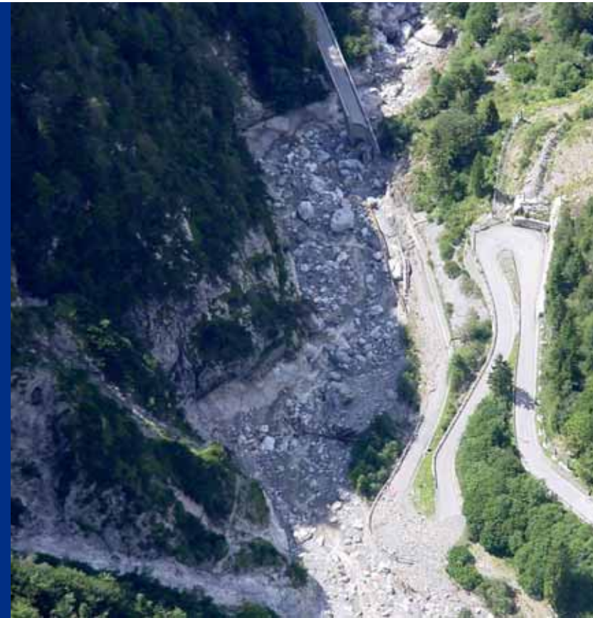
Before the intervention
