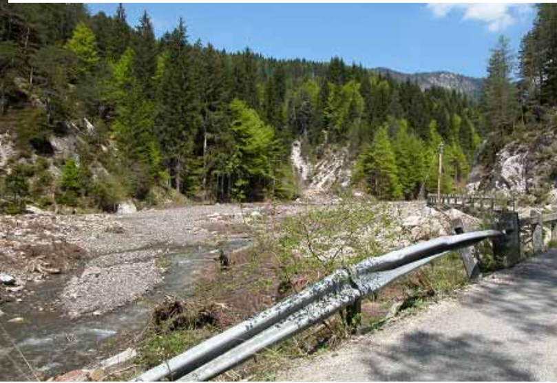
Before the intervention
