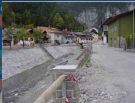
Gravel and material removal from the bed of the creek
