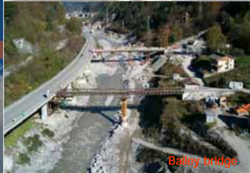
River side defenses and new bridge
