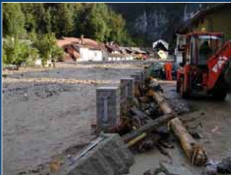
Gravel and material removal from the bed of the creek
