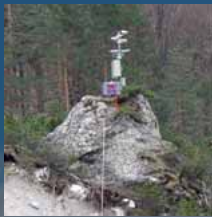
Cameras and laser-distancemeter connected in real-time to the operative center by means of radio-links, spread-spectrums and GPRS/GSM
